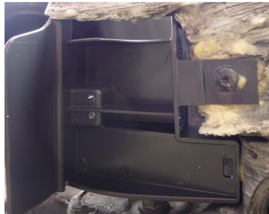
Figure 4 New adapter screw in the same position as before
